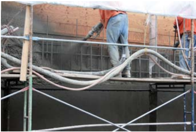
Bench gunning placement method
