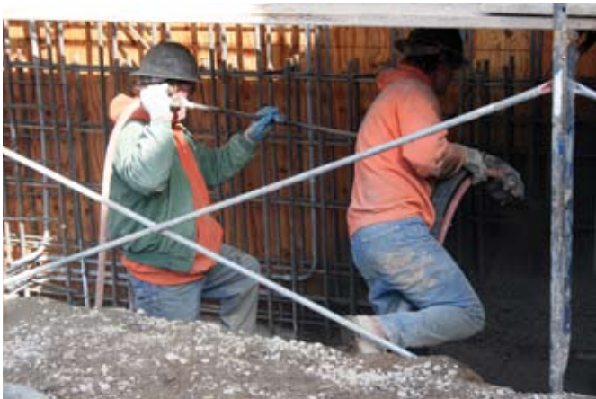
Bench gunning and blow-pipe operator
