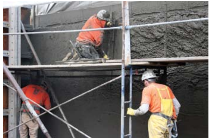
Cutting and finishing shotcrete wall
