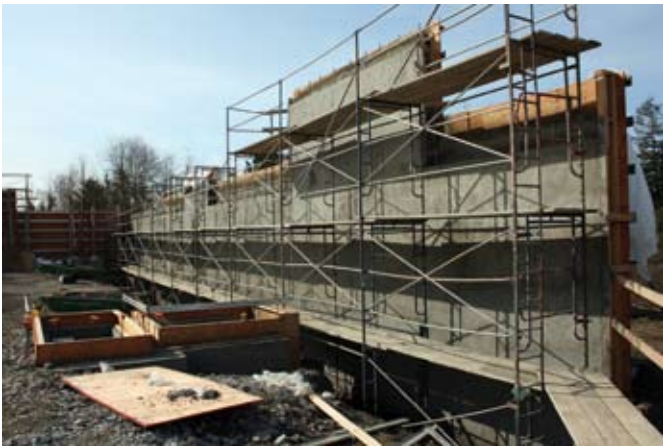
A completed wall
